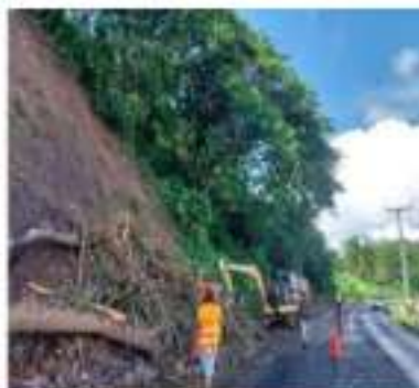
Figure 2 Shows clearing a landslide along the East Coast Road, where repeatedilly events continue to disrupt transport access
