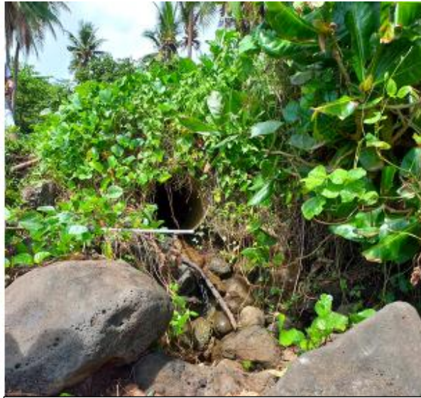
Road drainage culvert
