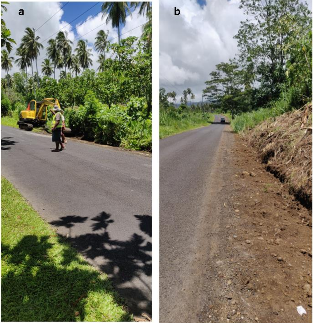
Figure 4.10 Road verge Clearance Under Operations (a) and Resultant Cleared Verge (b)
