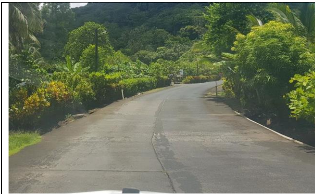
Plate 1: Concrete ford river crossing, ECR
