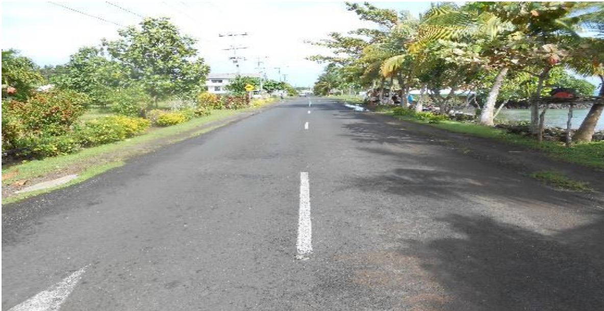
Photo 2.1: WCR – Present condition and proximity to the sea
