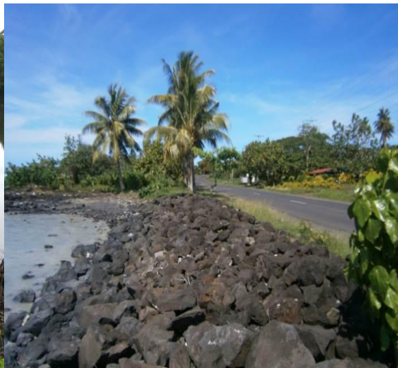
Photo 4.2: Seawall – WCR proximity to sea
