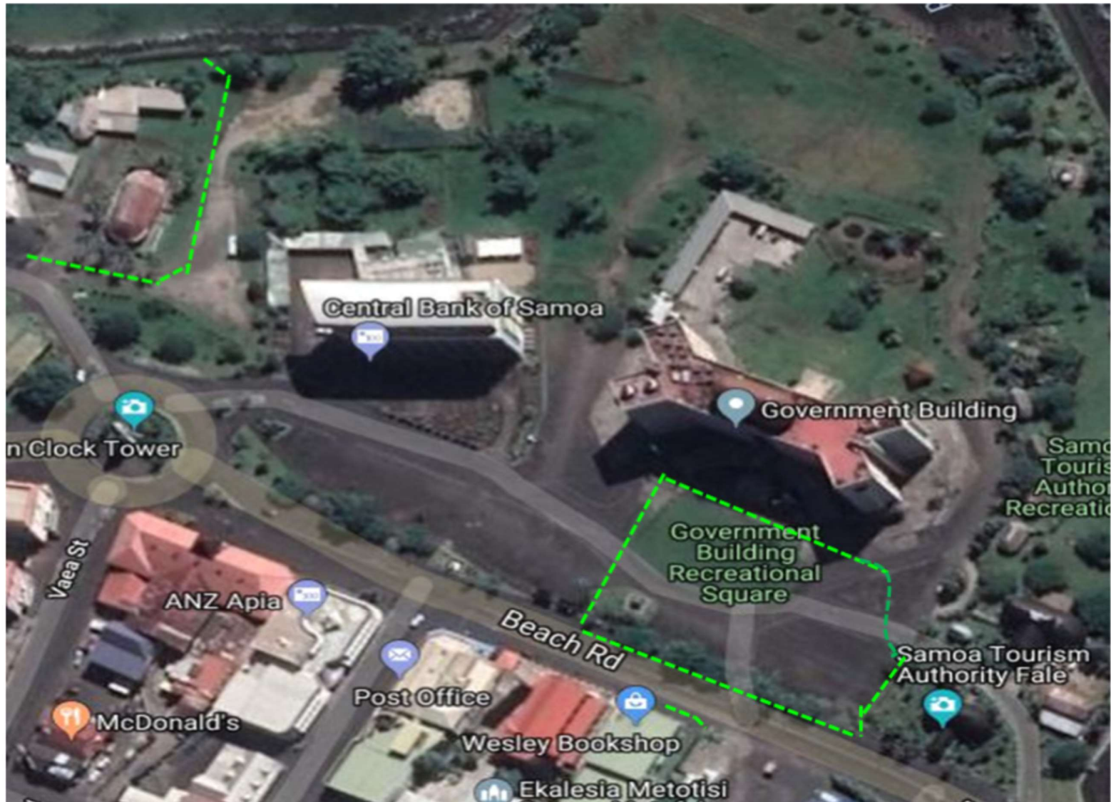
Green dotted lines show current restricted areas of the Central Apia Waterfront area undergoing construction.
